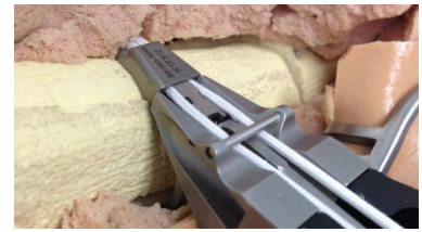
G. Engage nosepiece with clasp.
